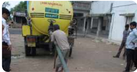
Desludging Services for On-Site Sanitation Systems
