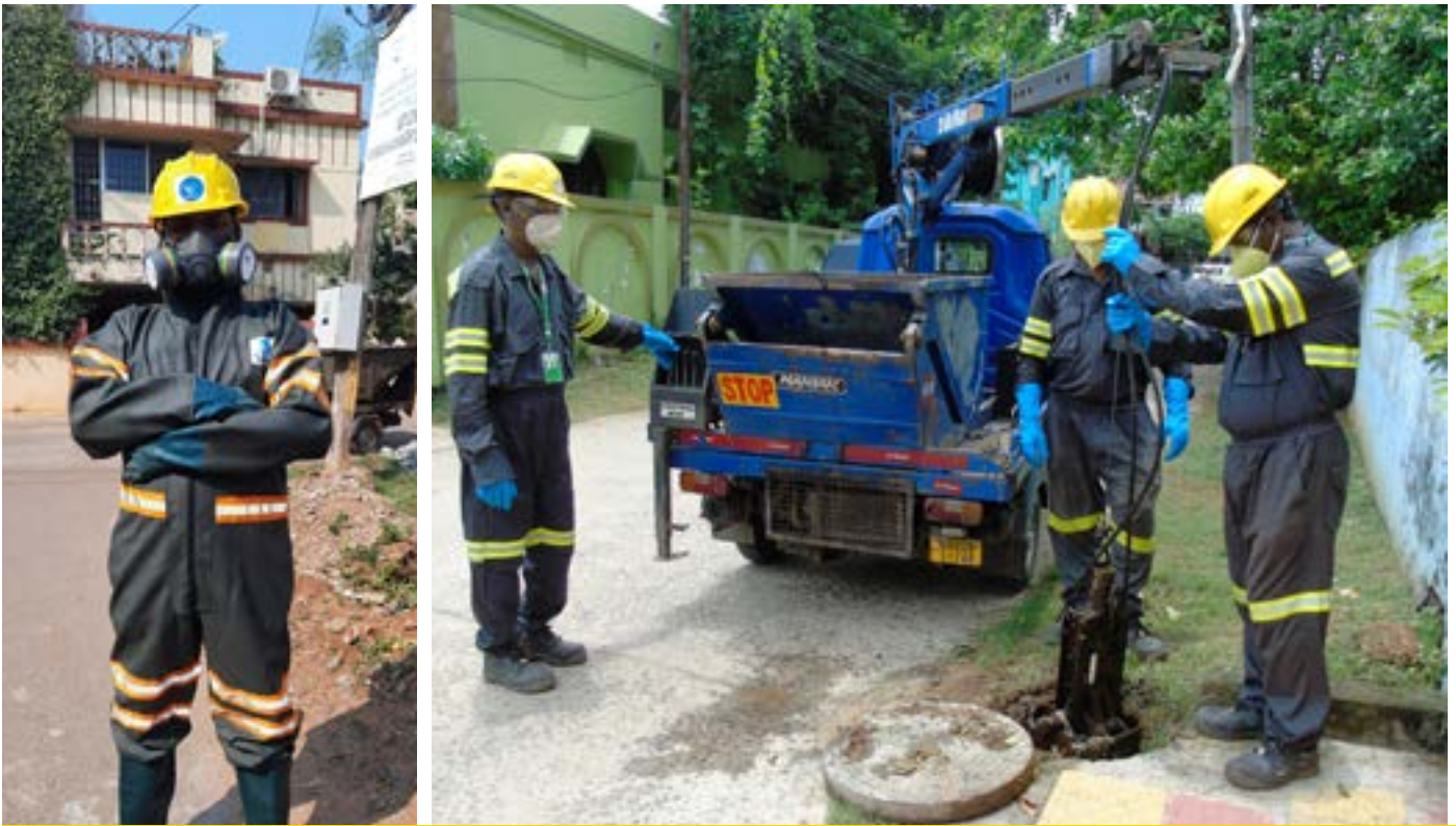
Trained and skilled workers engaged in cleaning of sewer line
