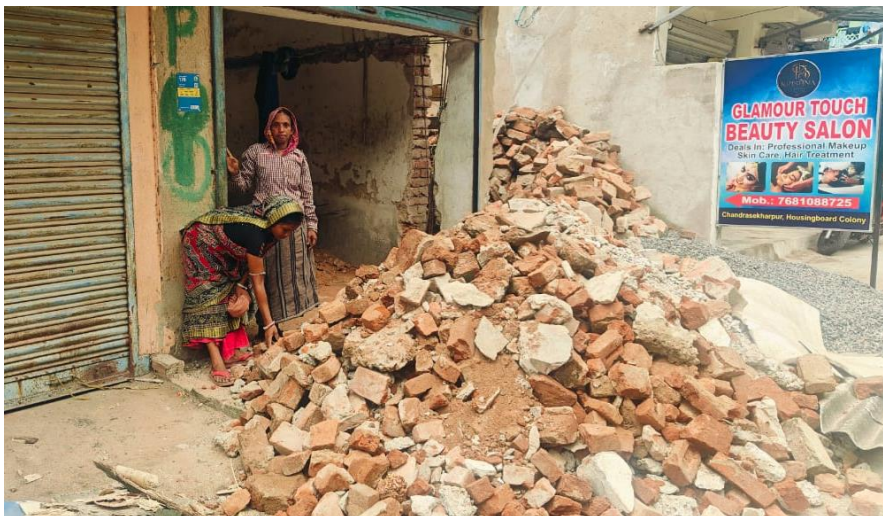
Women construction workers undertaking manual labour at an urban construction site
