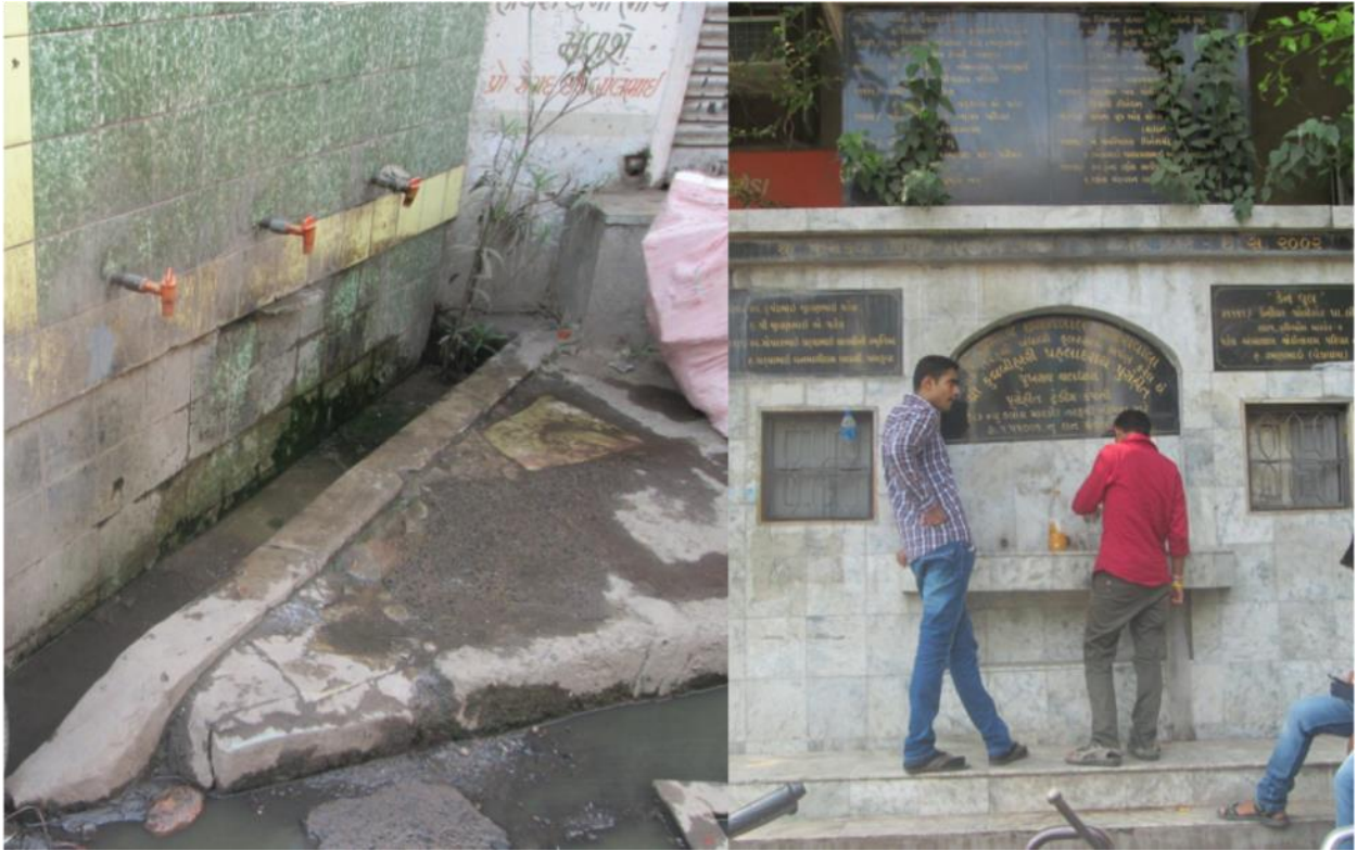
Drinking Water Facility at Panchkuva Market
