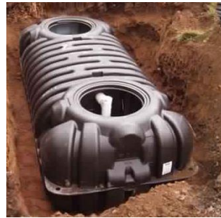
Placement of prefabricated tanks
