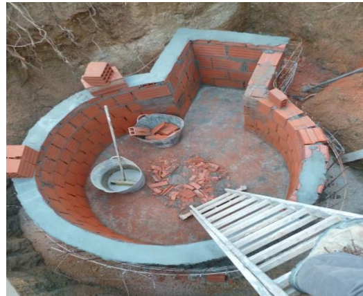
Circular design of Septic tank
