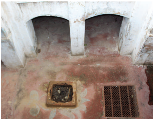
Slabs have filled in the openings on the lower level
