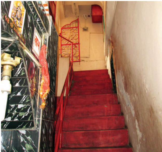
The residents have converted the entire structure
