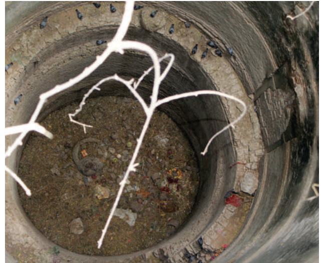
The water table is far below the original level
