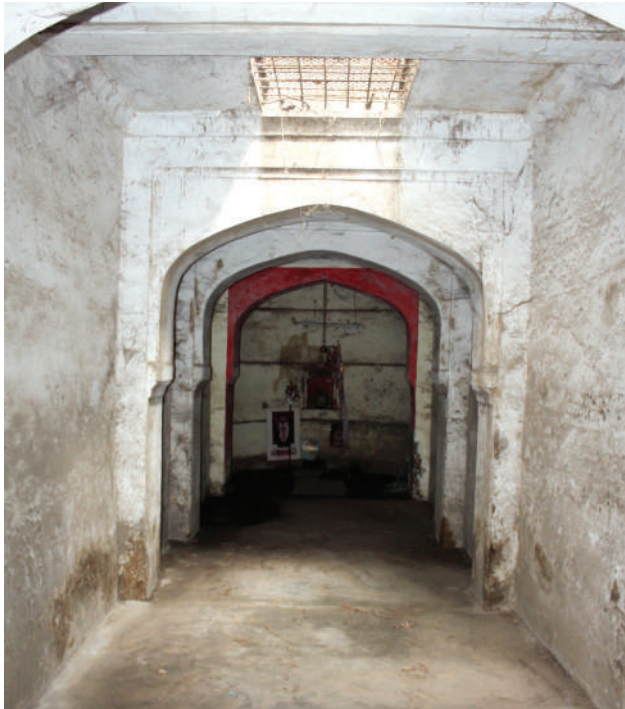
Slabs have been filled till the well shaft
