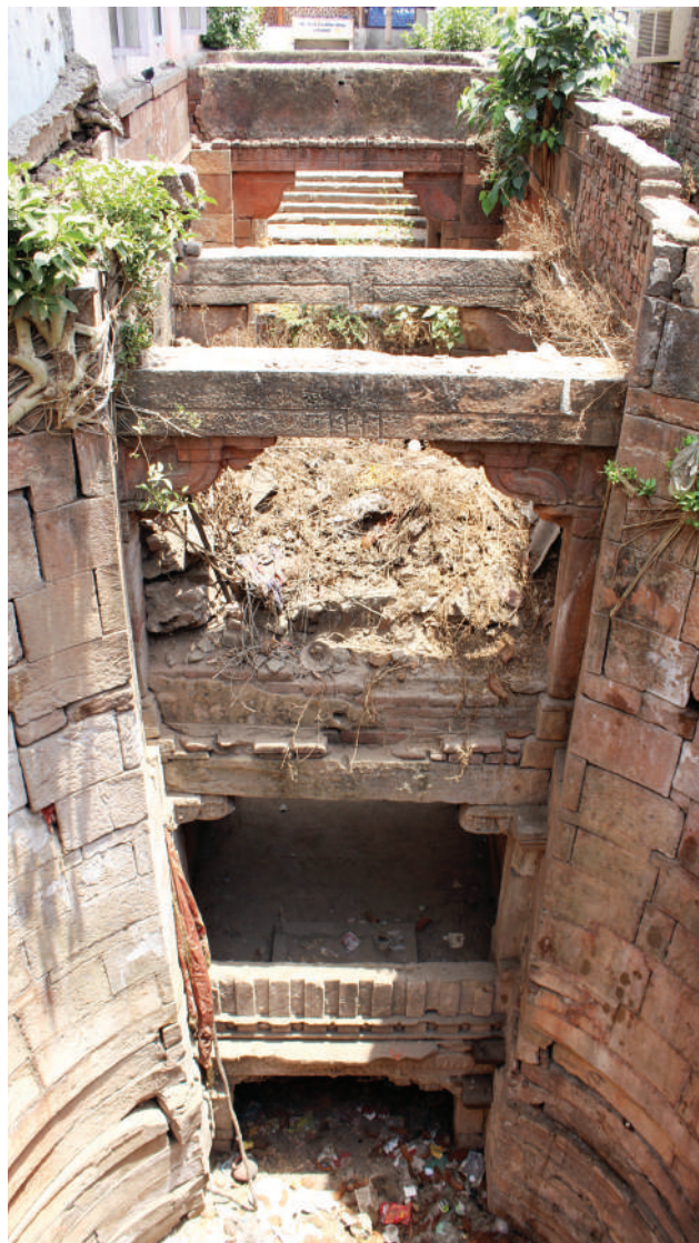
Kutas get narrower at lower levels
