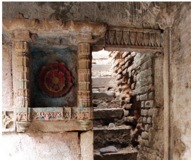
The niches have been carelessly painted
