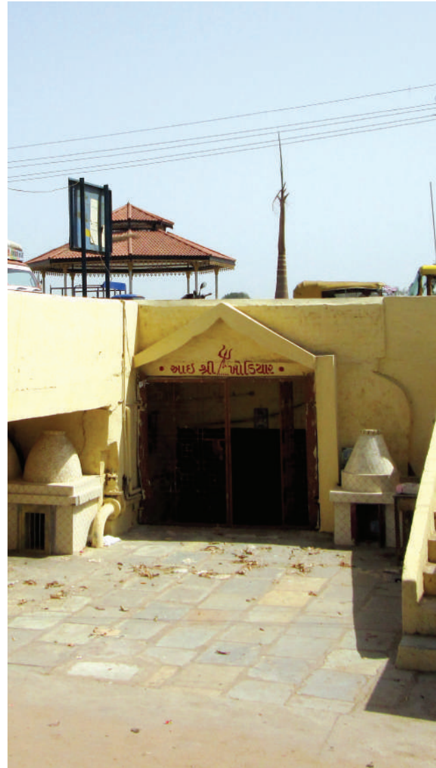
A road has been built over the well
