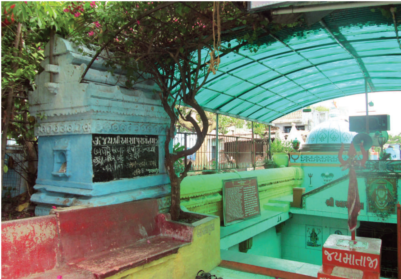
Stepwell has been insensitively renovated by the temple administration
