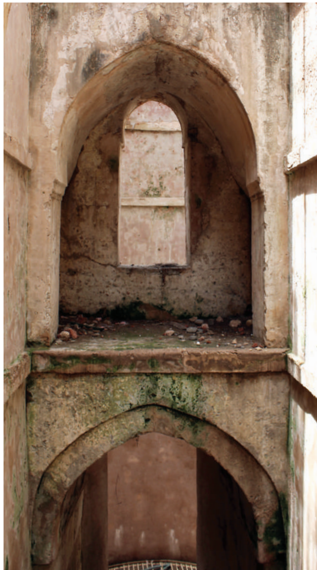
The change in material is clearly visible
