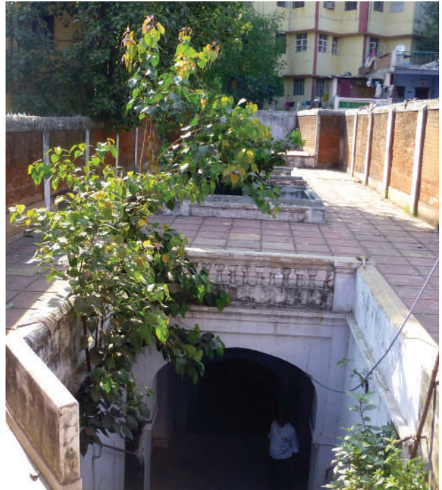
Toda at entrance have been removed
