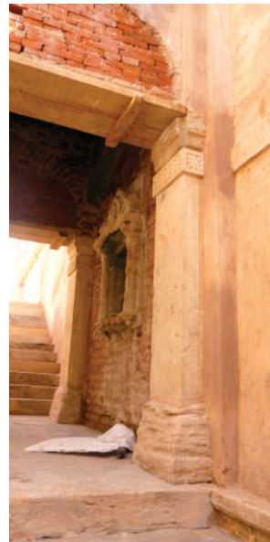
Columns during restoration
