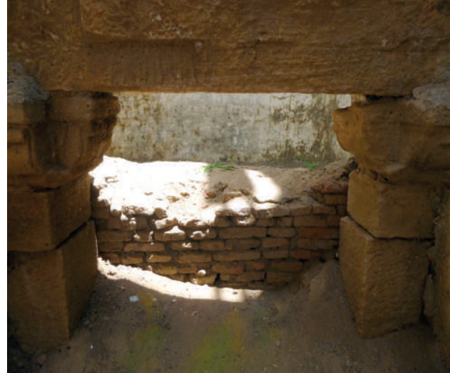
The beam and column system is visible
