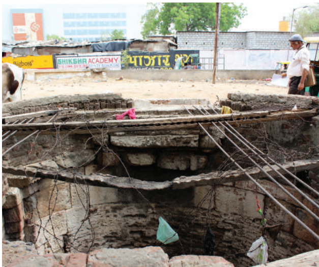
View at top of well shaft
