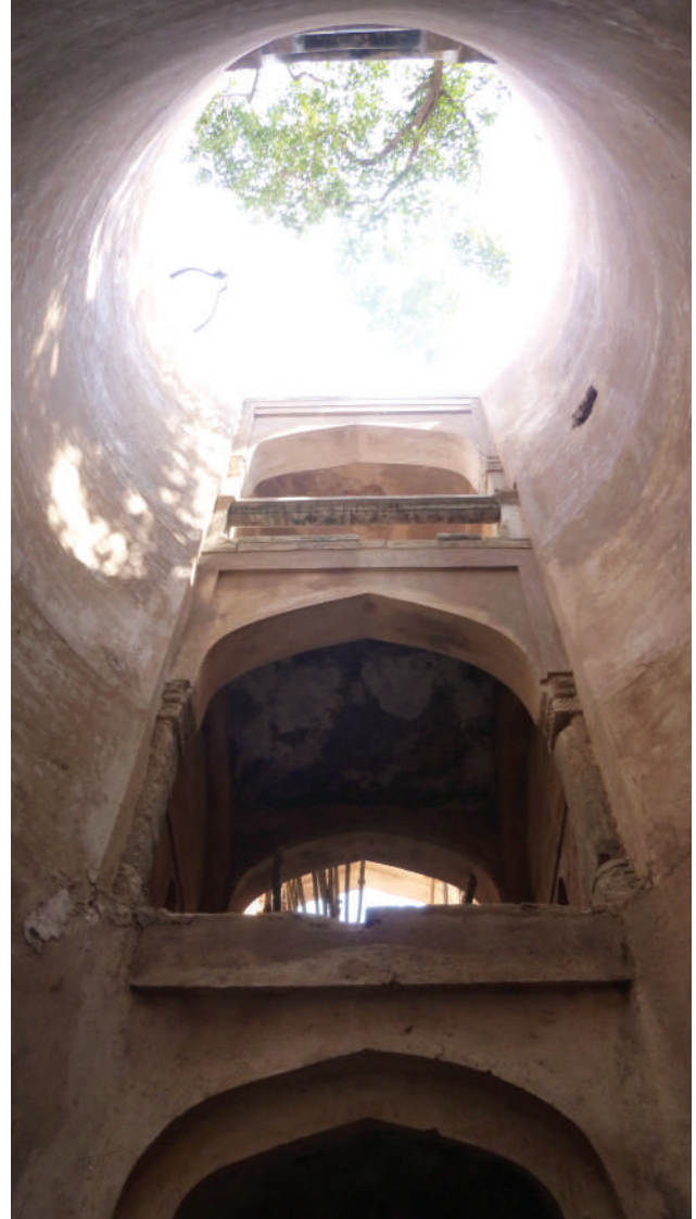
View inside well shaft
