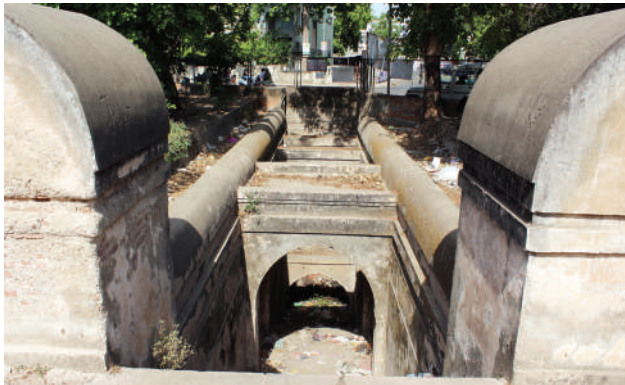
View towards well shaft
