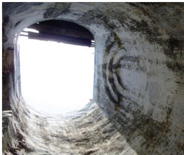
Layered arches are visible in the well shaft
