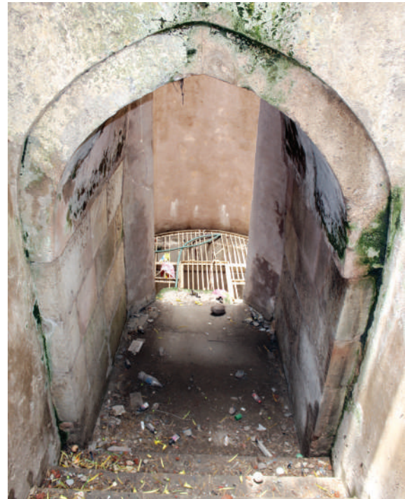
Stone is used in the lowest arch
