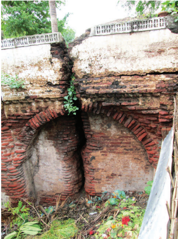
Brick arches are clearly visible in the side walls
