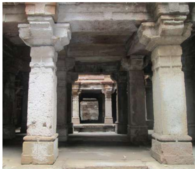
View along second floor
