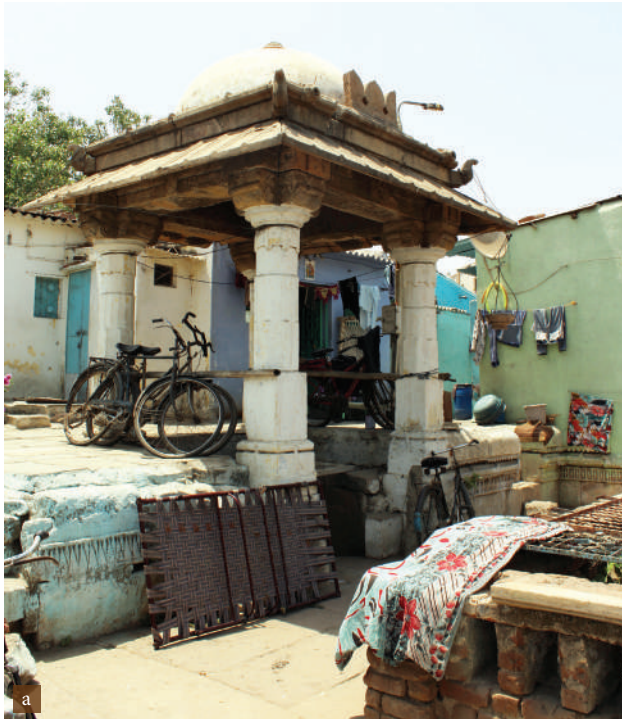
a. Dome over spiral staircase
