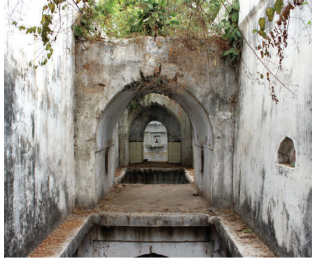
The structure has been recently covered with cement plaster
