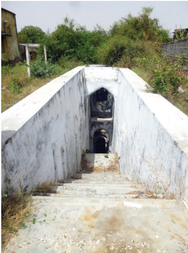
Cement plaster and paint have been used to restore this well
