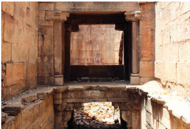
View of the well shaft
