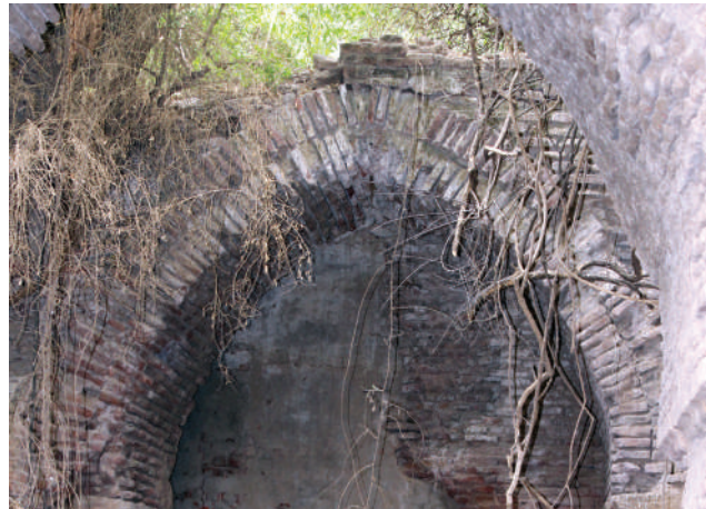
The brick masonry in the arches is clearly visible
