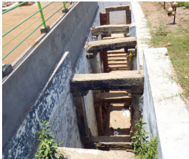
The stepwell uses a system of stone beams and columns
