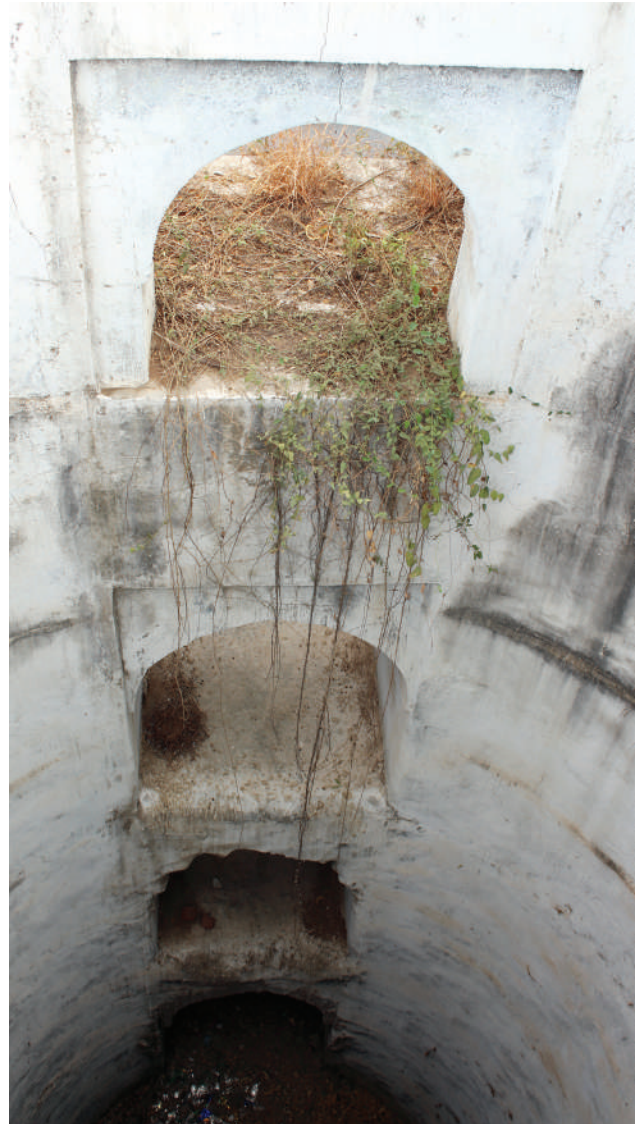
The well shaft is still accessible
