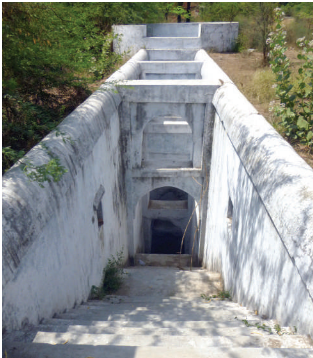
The structure has a combination of beam, columns and arches
