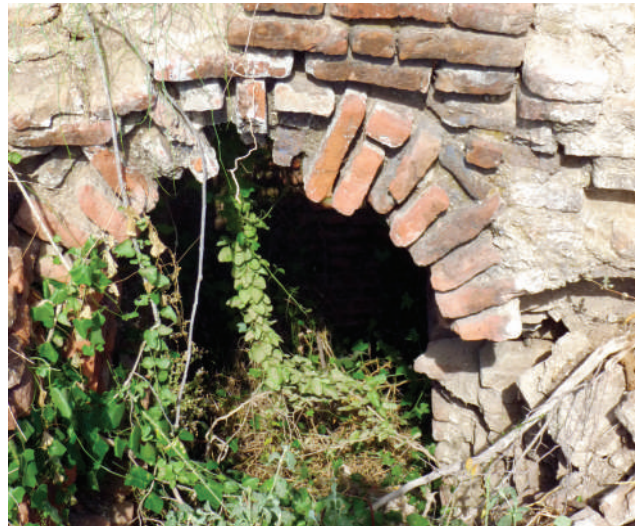
Narrow brick arches are visible along the length
