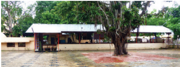
A steel roof has been erected over the stepwell
