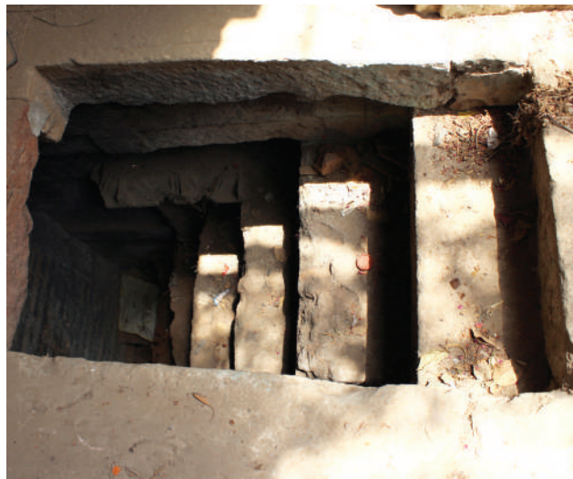
Steps have been cut out in the floor slabs
