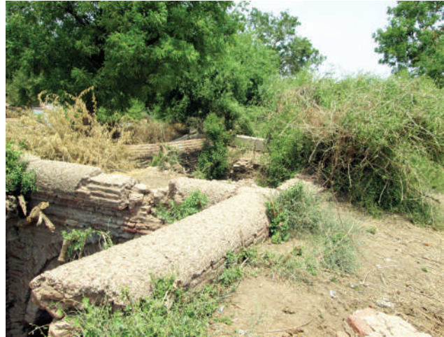
The well has almost been filled up
