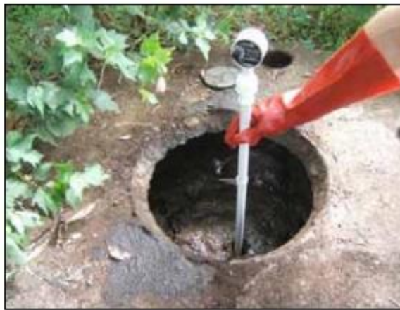
Fig. 2.7.2: Checking the sludge in the septic tank
