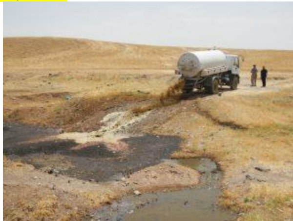
Fig. 2.7.8: Empty the sludge tank
