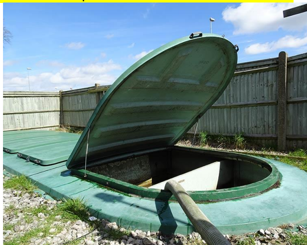
Fig. 2.7.9: Cover the septic tank
