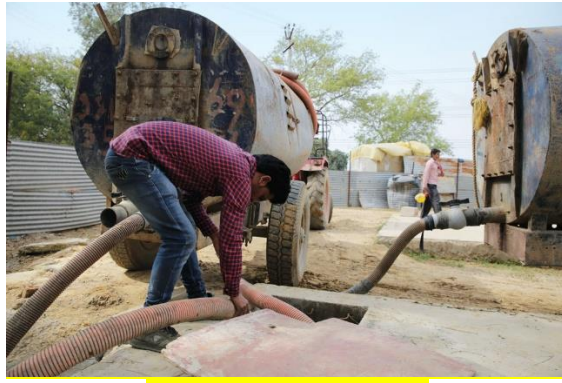
Fig. 2.7.7: Install suction pipe
