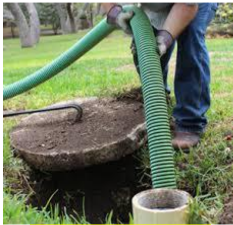
Fig. 2.7.5: Uninstall the suction pipes
