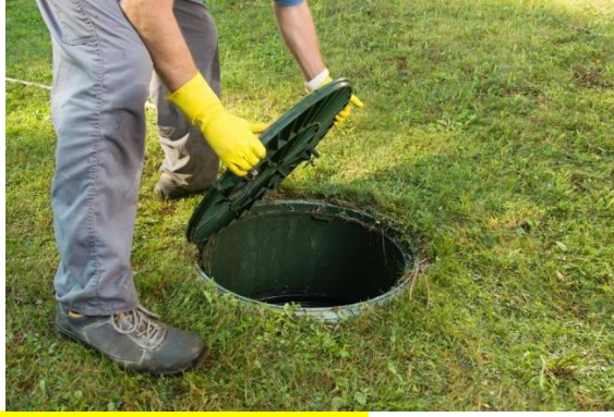
Fig. 2.7.4: Closing the access cover
