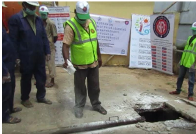
STEP 7: Add chlorine on hose after emptying
