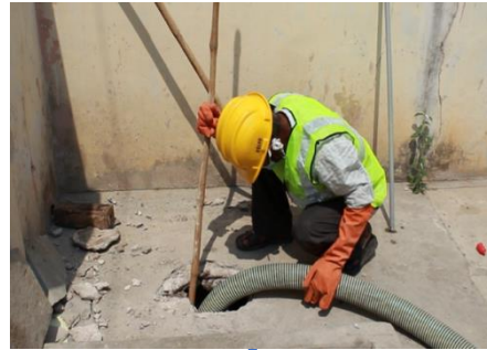
Check the consistency of sludge
