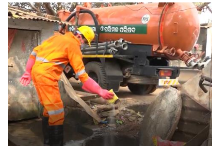
Add chlorine in the septic tank
