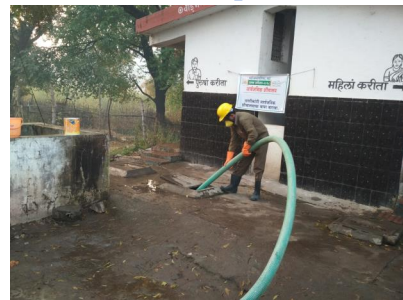
Install hose in septic tank
