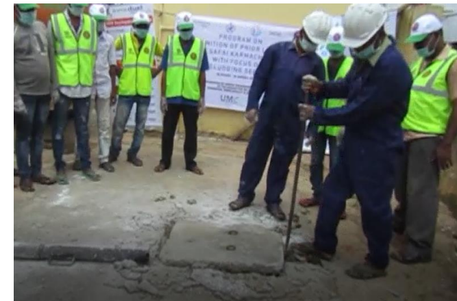
STEP 8: Close the lids of septic tank
