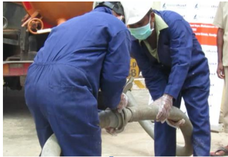
Connect hose pipe to septic tank
