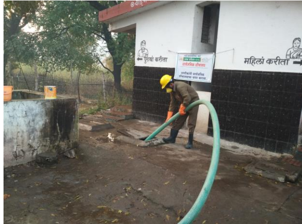
STEP 1: Install hose in septic tank
