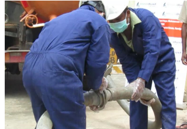
STEP 4: Connect hose pipe to septic tank
