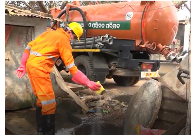
STEP 2: Add chlorine in the septic tank
