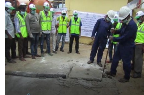
Close the lids of septic tank
