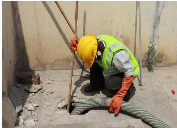
STEP 3: Check the consistency of sludge
