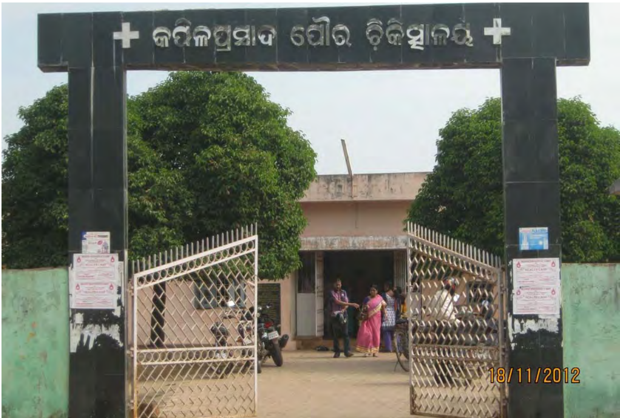
Photograph 16 Most dispensaries in the city are in fair condition but need some up gradation
