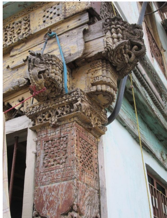
Figure 13 Beam head and column capital at a house, Kudasan
