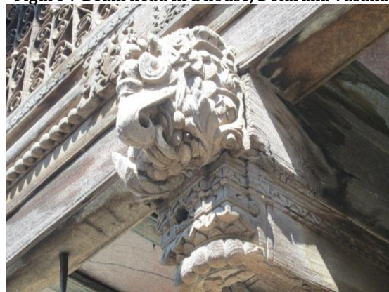
Figure 7 Beam head in a house, Dolarana Vasana
