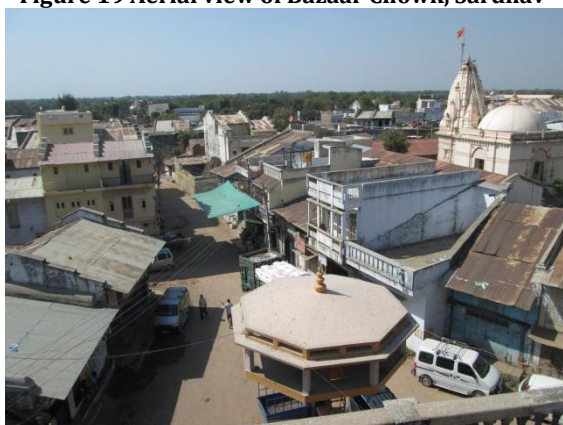
Figure 19 Aerial view of Bazaar Chowk, Sardhav
