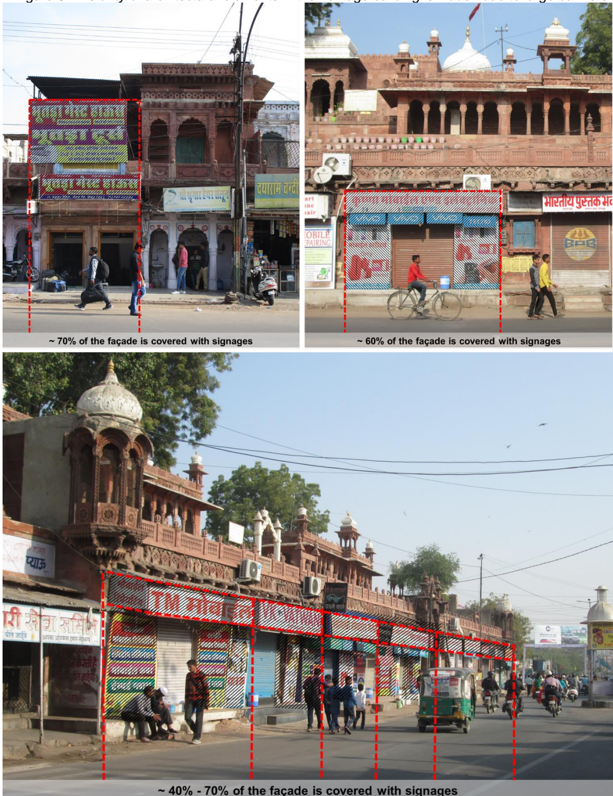
Figure 34 Visibility of architectural elements in the heritage building is hidden due to large banners
