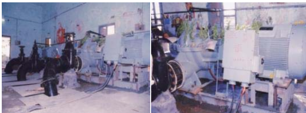
Sarkadia Pumping Station
