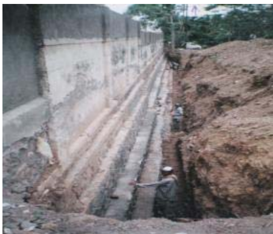
Repair work in progress
