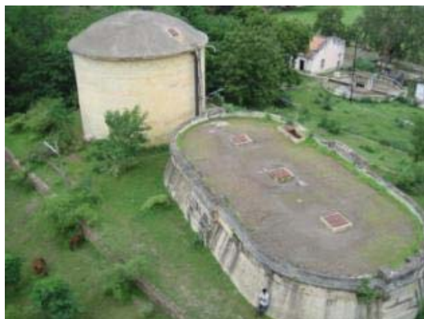
Storage Tank at the Filter Plant
