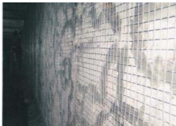
Wire meshing as Reinforcement
