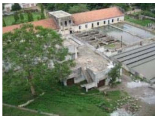
Takhteshwar filter plant
