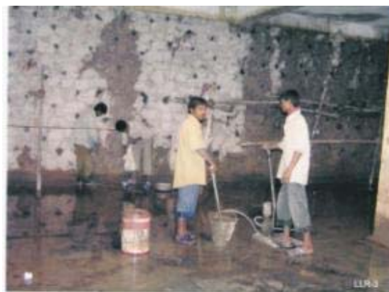
Repairing and cleaning of the Water Tank 1
