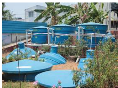
Biogas plants for processing organic waste; L- Model biogas plant for managing kitchen waste R-Temple Green initiative
