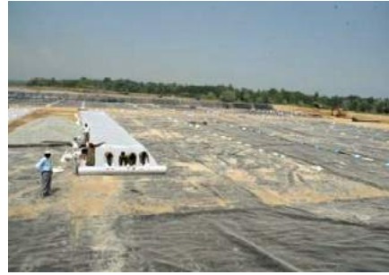
Overlaying the HDPE Liner
