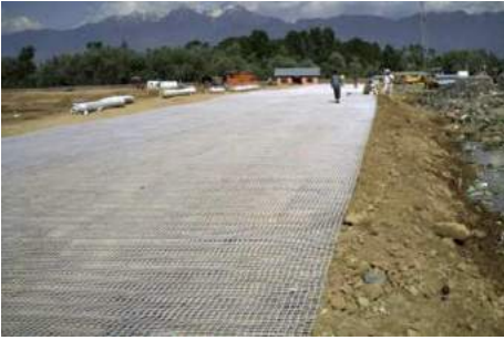
Laying of geogrid
