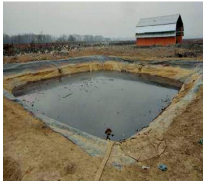
Leachate collection pond
