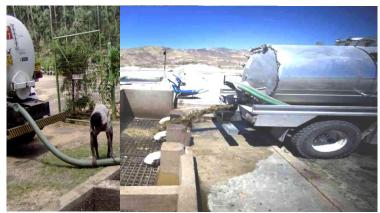
Figure 13 Sludge disposal into inlet chamber of STP Image Source: septage management guide for local governments, 2007, David M. Robbins
