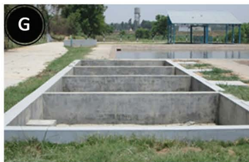
Sludge Drying Bed
