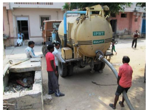
Figure 3 De-sludging septic tanks from residential areas
