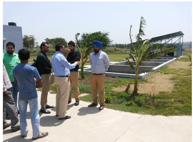
Below: Site visit with ULB officials at small bore sewer system
